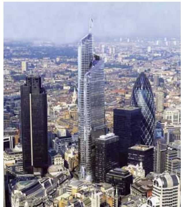
■ Bishopsgate Tower, Лондон
